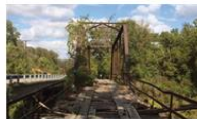
Decking damage: May 2015 flood
