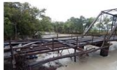
Decking damage: October 2015 flood
